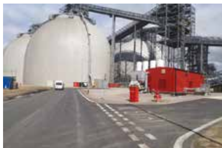
Power Station and Leeds University's School of Chemistry.
